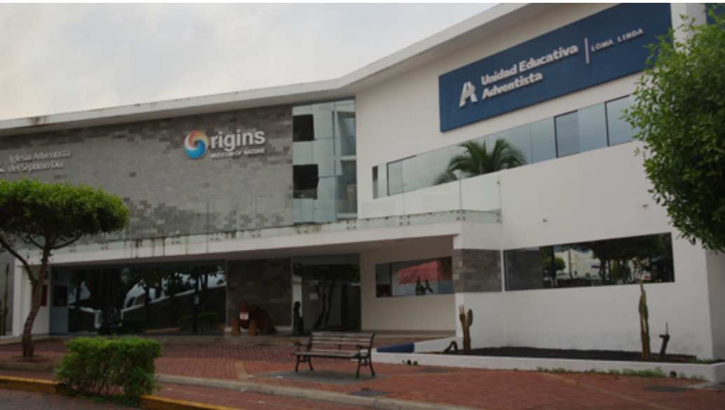
The building as seen from Charles Darwin Avenue housing the Origins Museum of Nature, the Loma Linda Adventist Education Unit, and the Seventh-Day Adventist Church.
